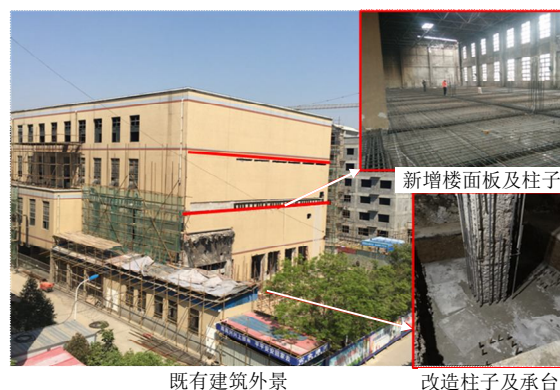
图 1 既有建筑及重点改造部位实物图 Fig.1 Photos of existing building and the reconstruction parts
